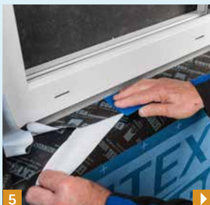
5 Seal the window joints on the inside and outside using CONTEGA.
