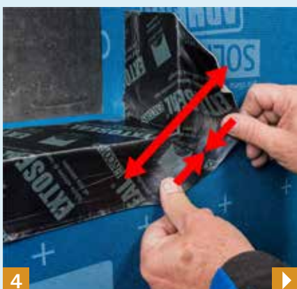
4 Form the sub-sill flashing using EXTOSEAL ENCORS.
