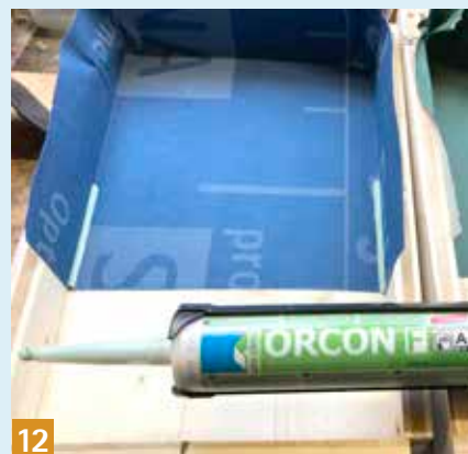
12 Additionally seal membrane overlaps at protruding walls using ORCON F.
