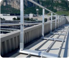
Railing anchored to the base by fusing
